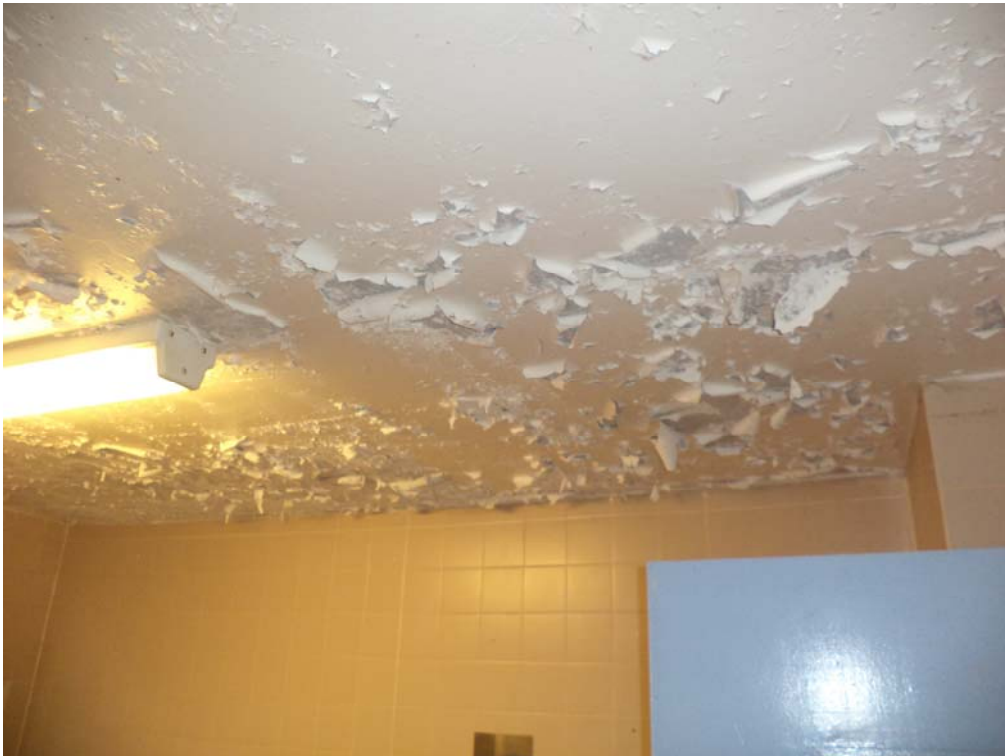
Paint peeling from the ceiling in a shower area on the closed site
