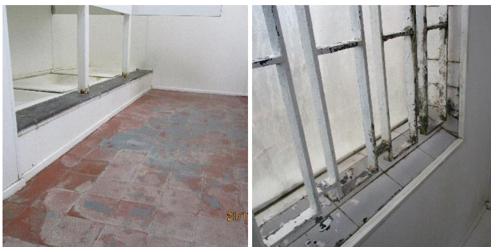
Floor and window in the shower room
