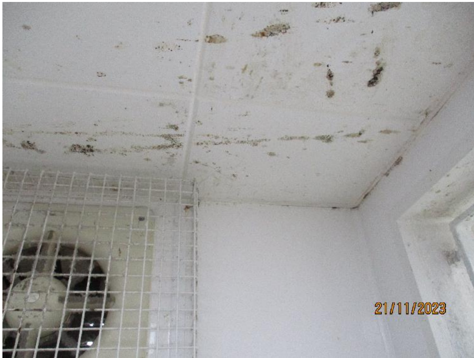
Shower room ceiling
