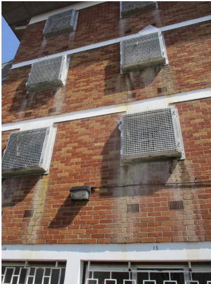
Stains beneath window grills on B wing
