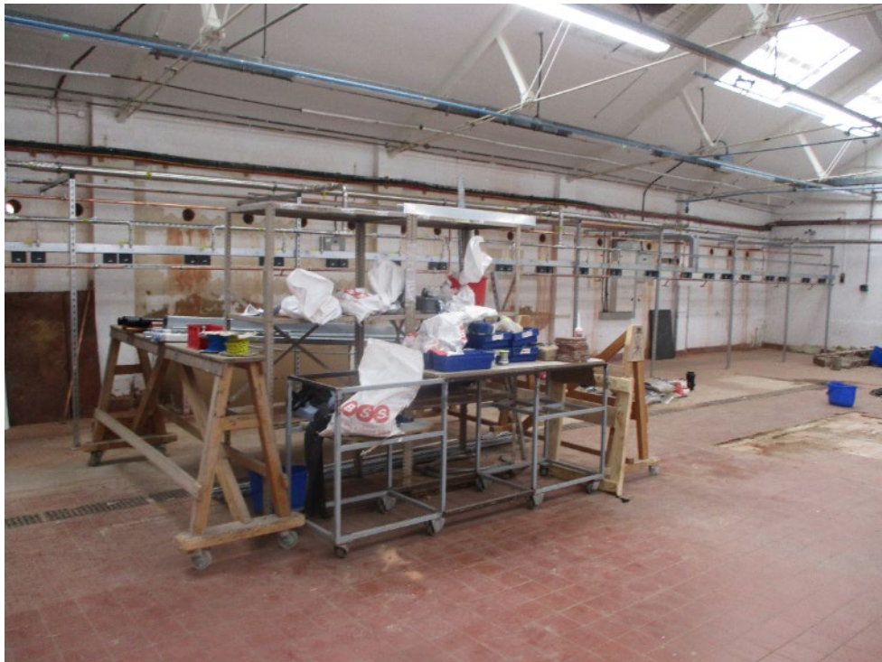
New laundry under construction
