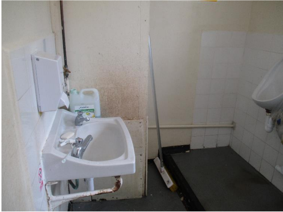
E unit toilet area
