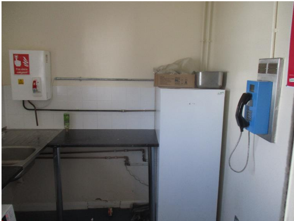
Telephone in kitchen area
