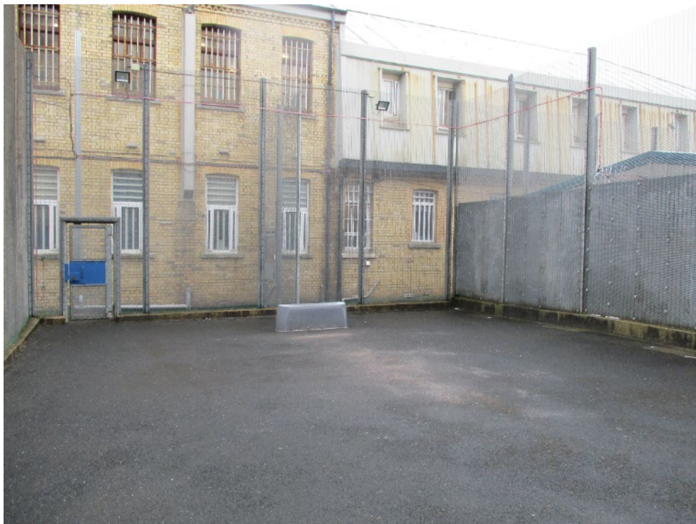
CEG exercise yard
