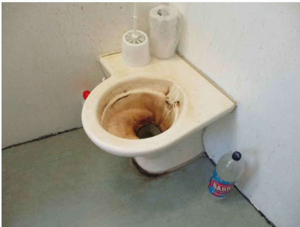
Toilet on M wing
