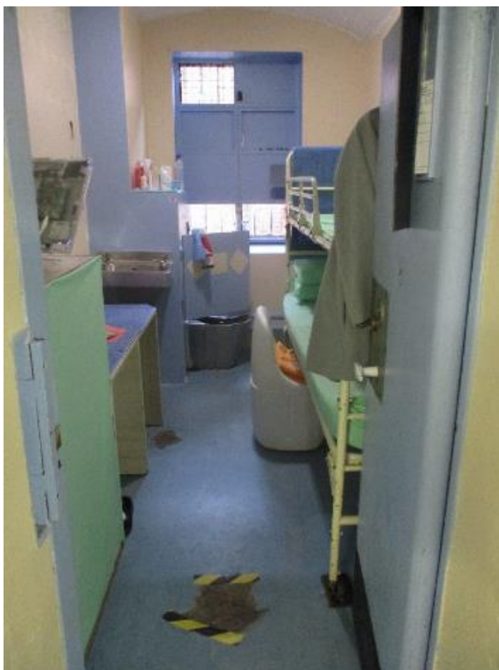
Cell with damaged window and floor
