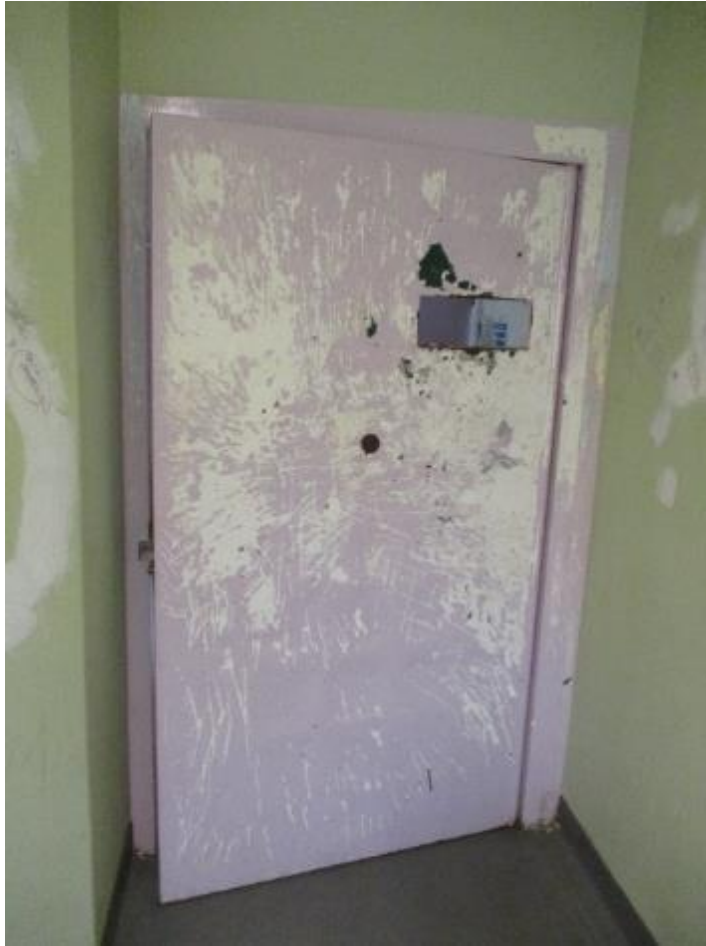
Back of a cell door on residential unit 4
