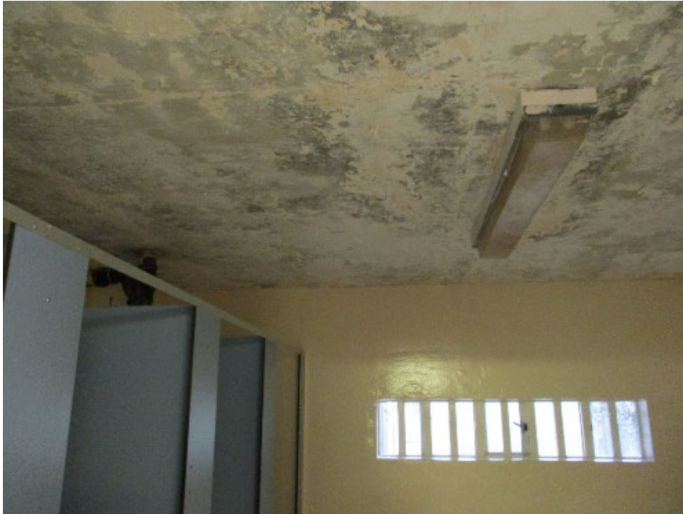
Shower room ceiling
