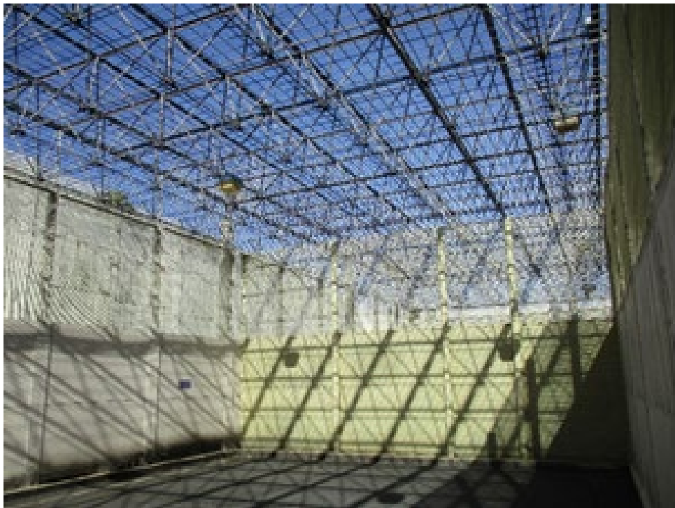
Segregation exercise yard
