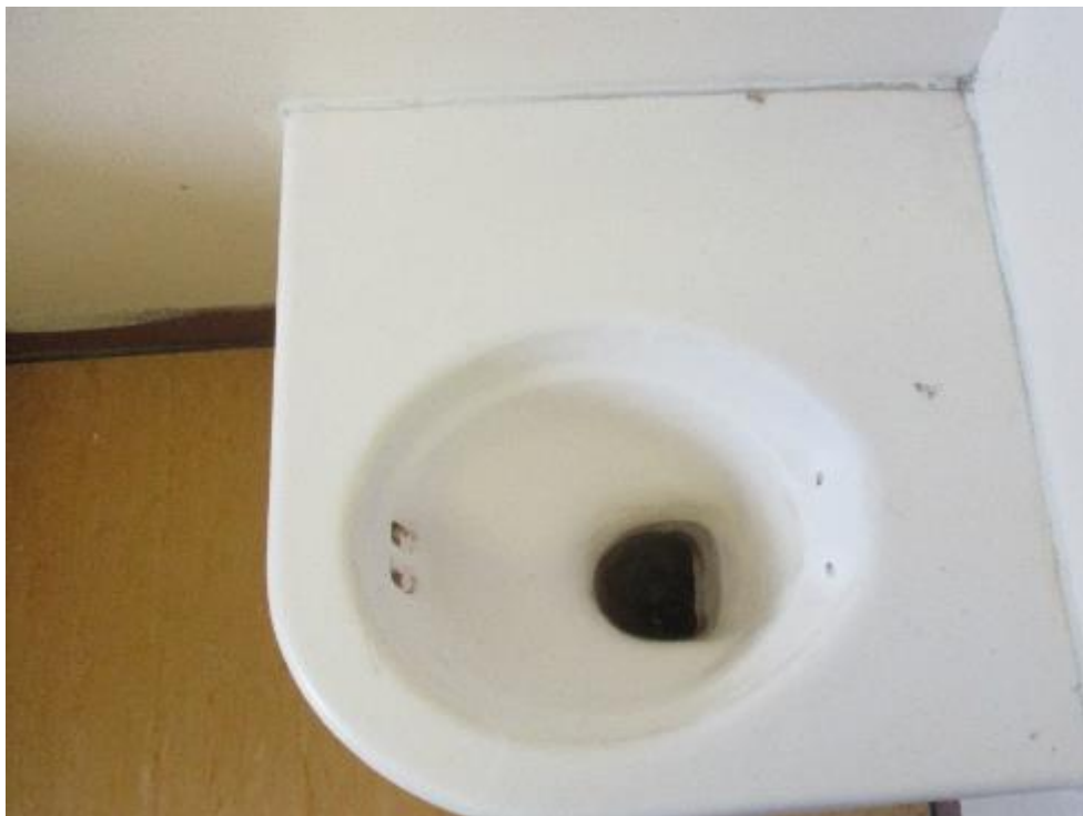
Toilets before and after specialist cleaning
