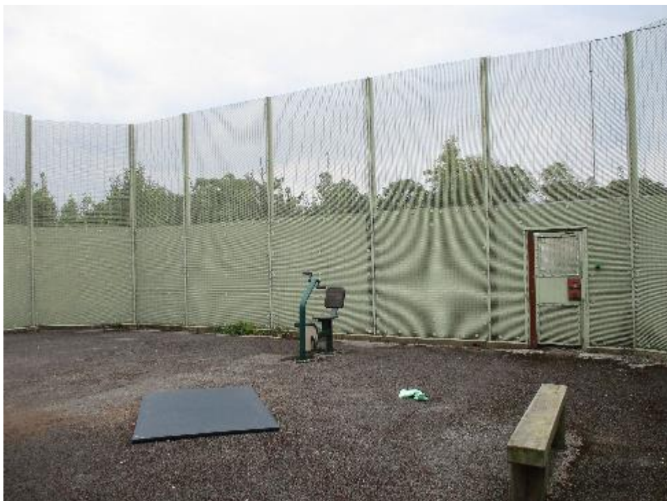
Segregation exercise yard
