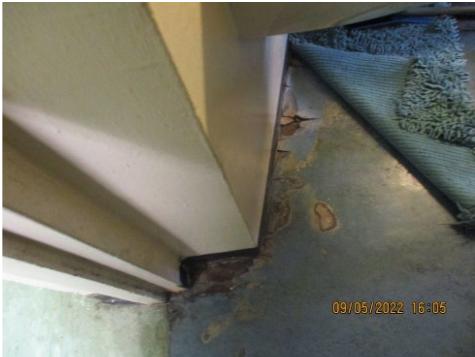
Damaged flooring in a cell
