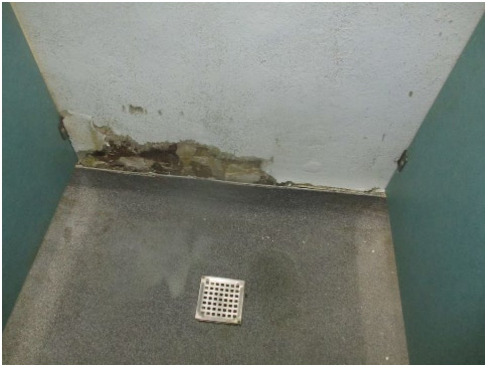
Shower wall on the category C site
