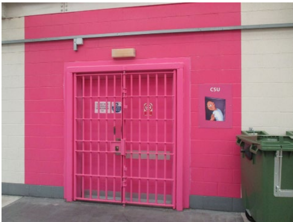
Segregation unit entrance
