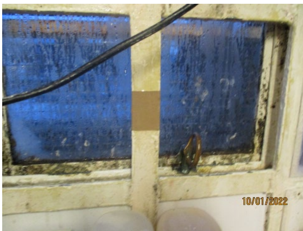
D wing cell windows
