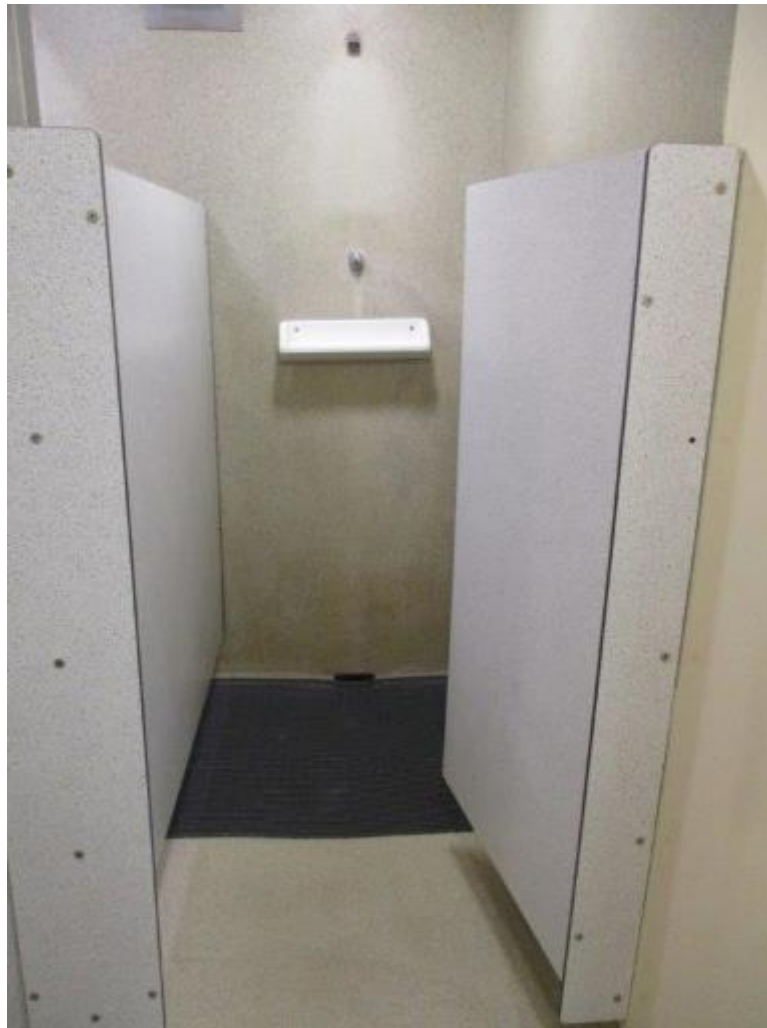
Shower on a residential wing
