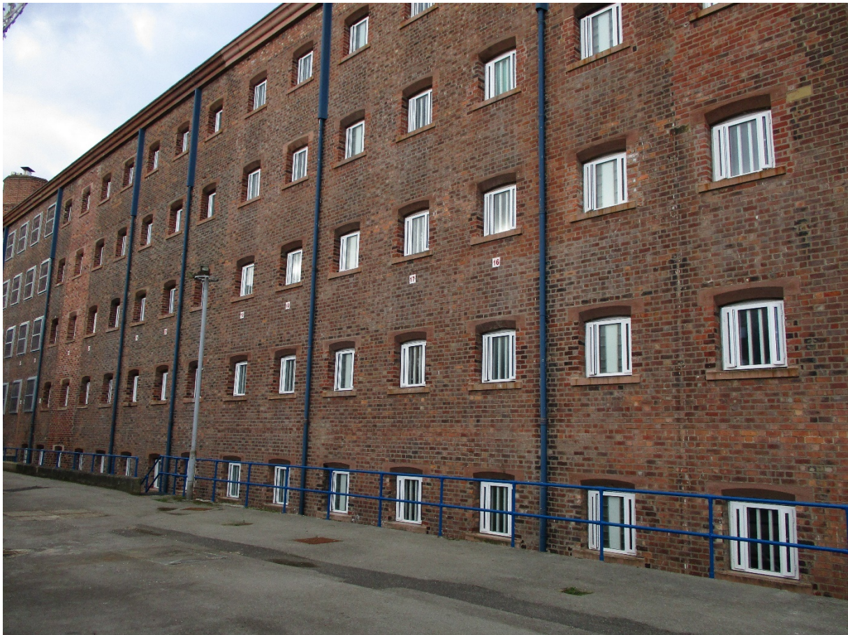
F Wing windows after refurbishment
