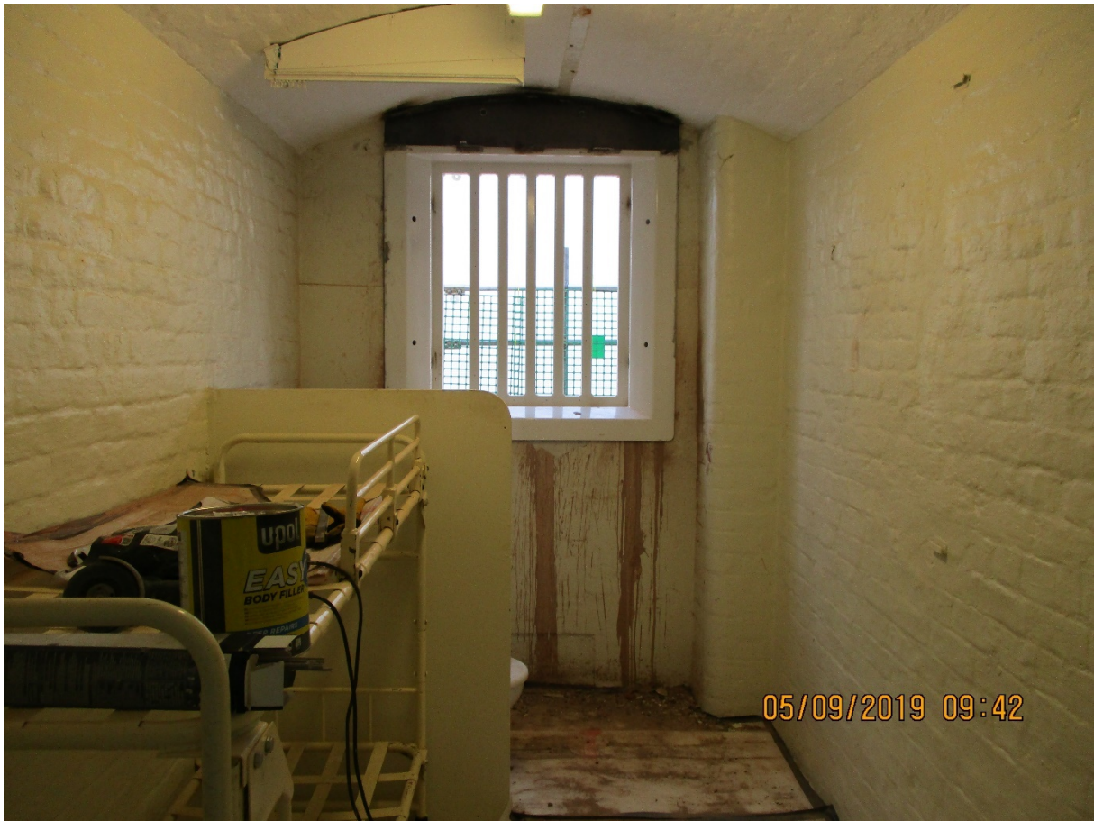
H Wing replacement window in progress
