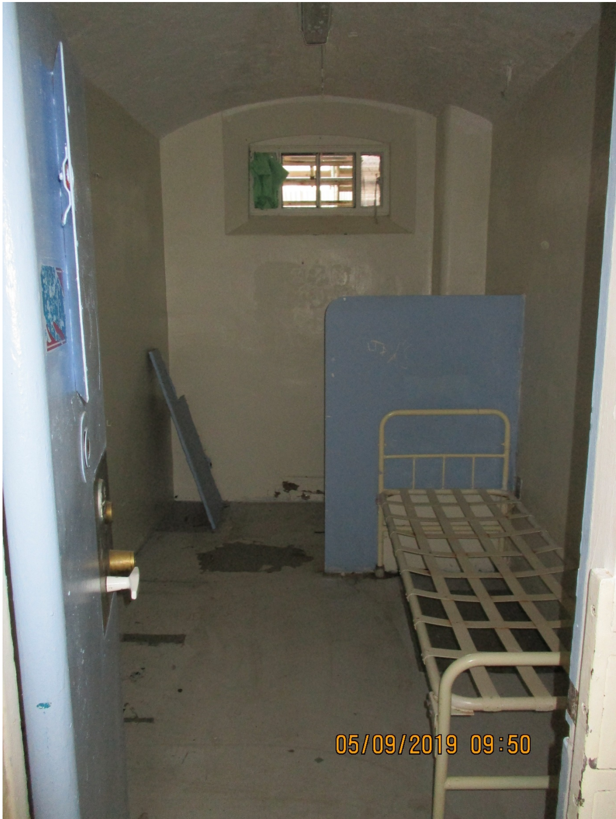
Victorian window prior to refurbishment
