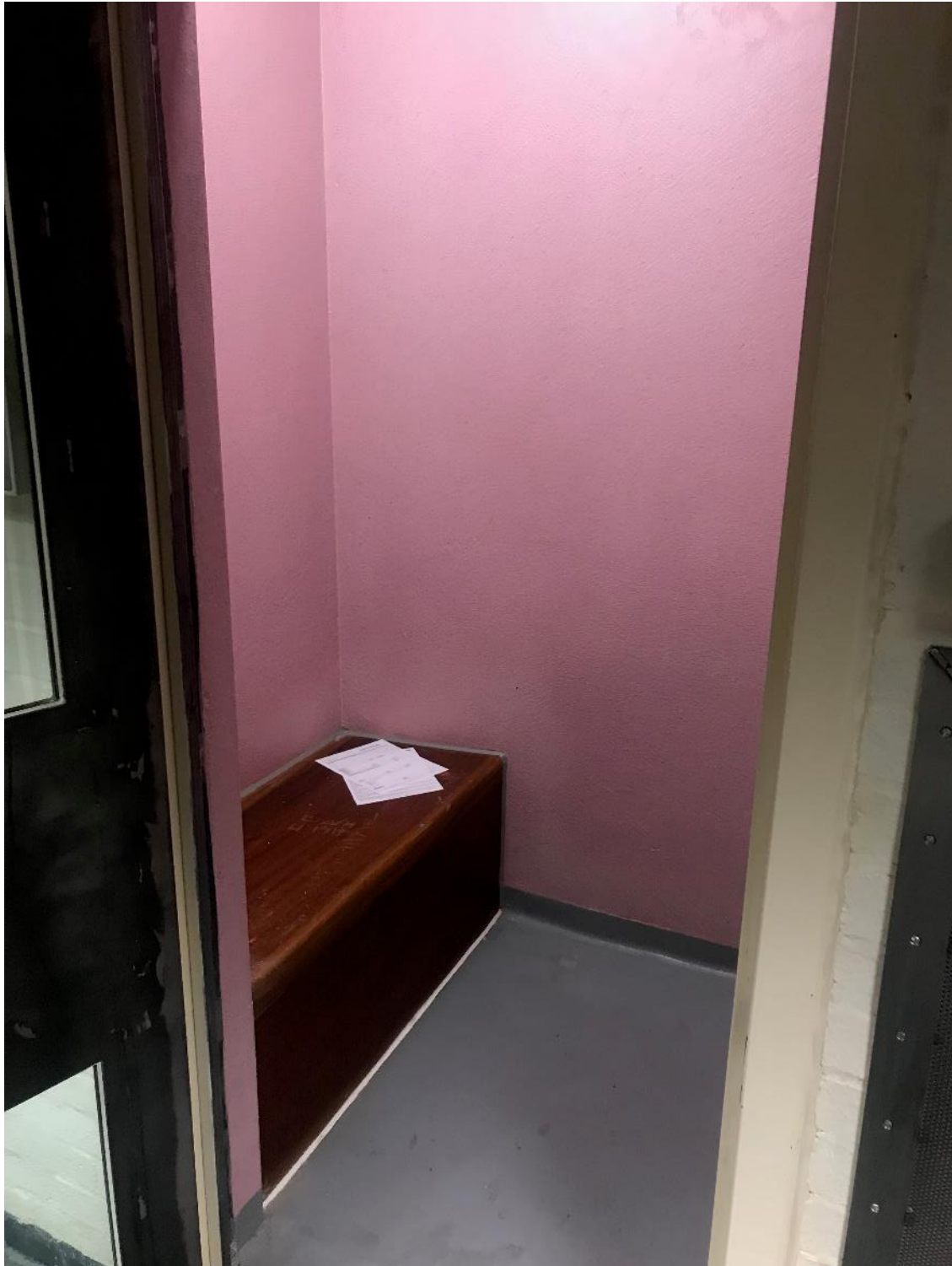
Small cell at Winchester Combined Court.
