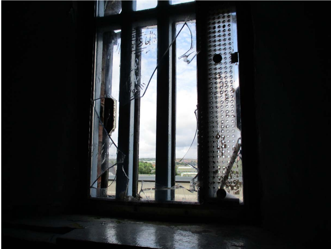
Photograph 3. Smashed windows with jagged glass
