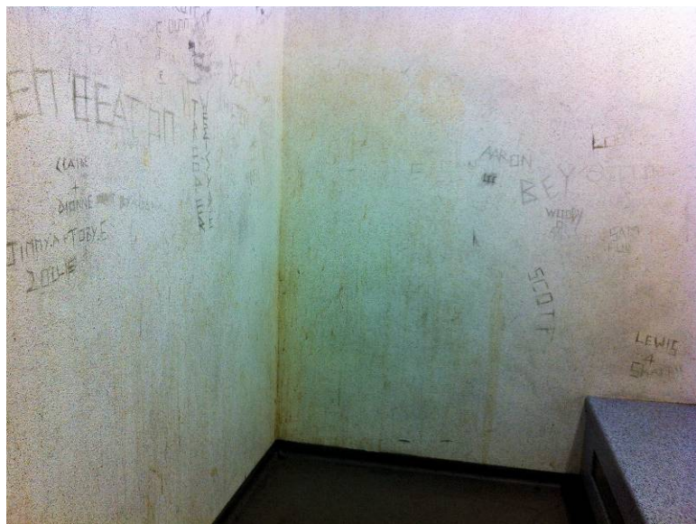
Cell wall, floor and bench at Maidstone Magistrates' Court
