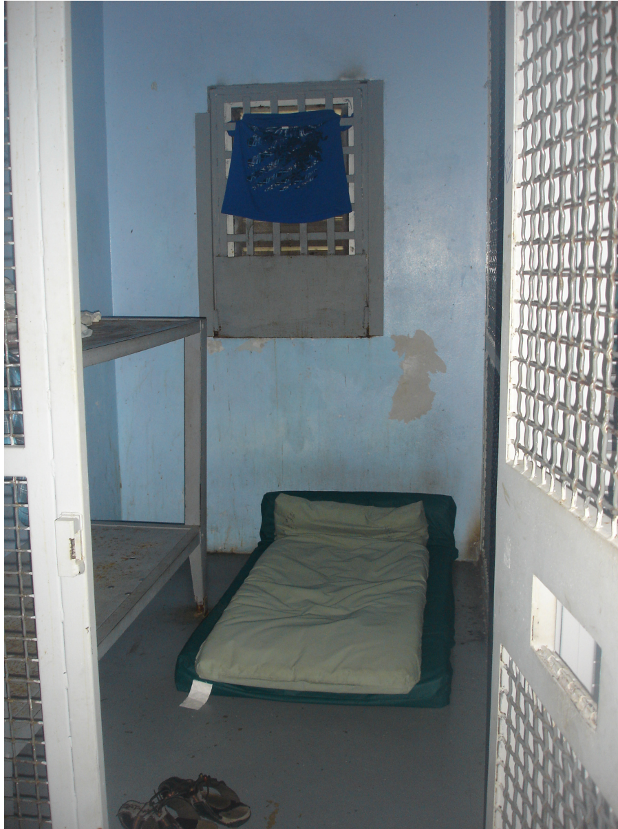
Cell in George Town police station
